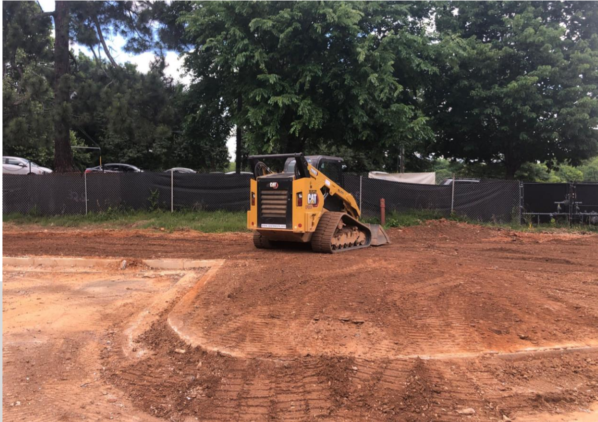
Final Grading Around New Addition Parking Lot
