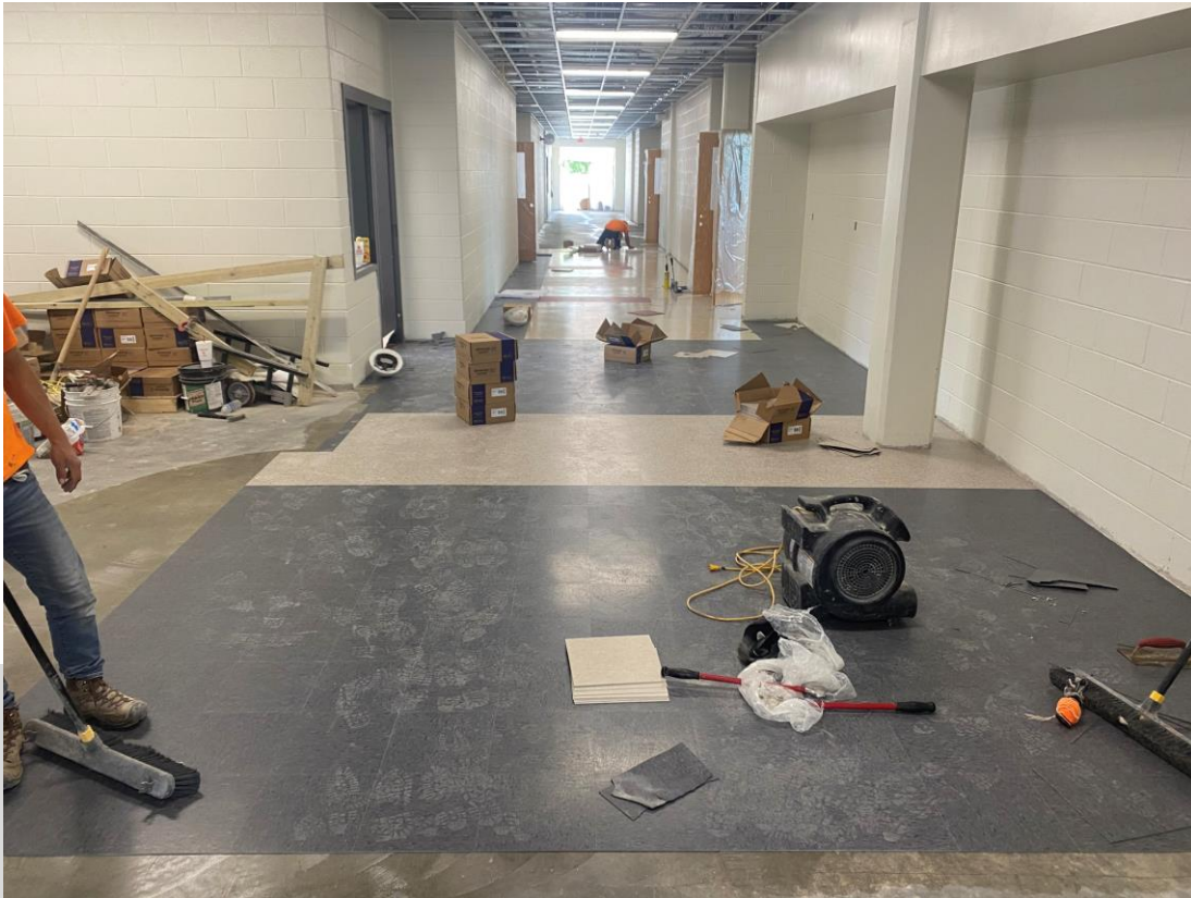
VCT Installed in Corridors of New Addition Building
