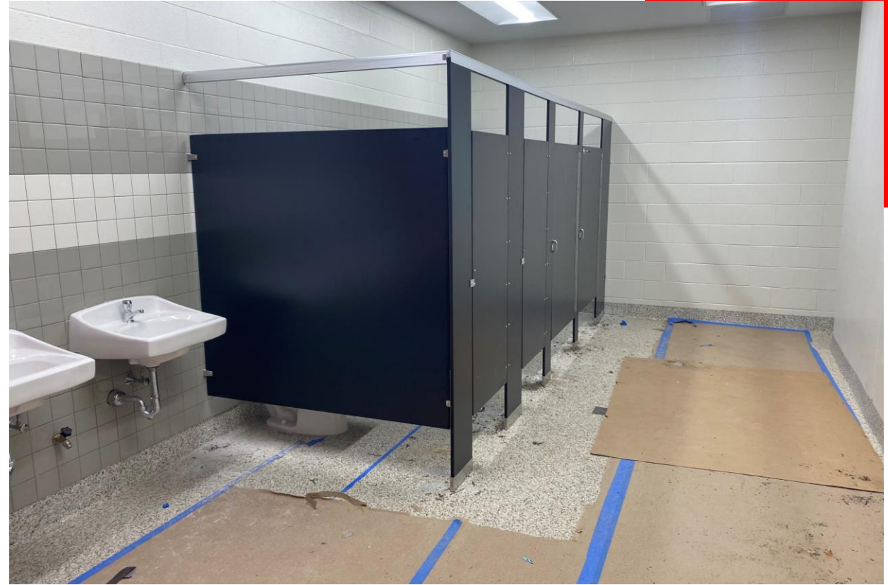
Toilet Partitions Installed in New Addition Building Restrooms
