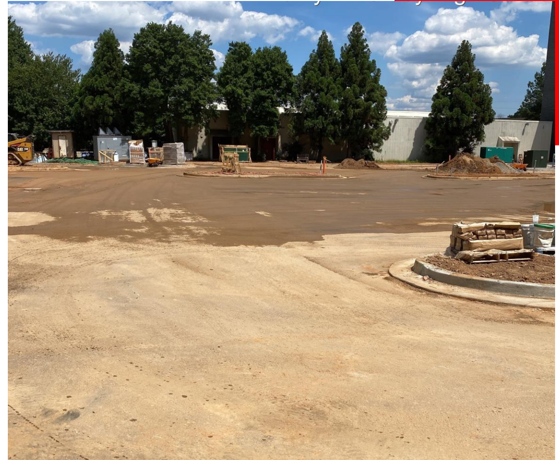
New Addition Parking Lot Cleaned and Ready for Topcoat and Striping Next Week
